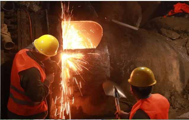
昼夜奋战铺设供水主管
